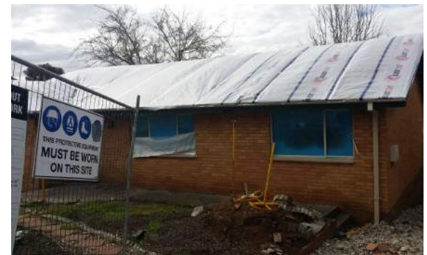
Asbestos Removal – Canberra, Australia (Authors Own)
