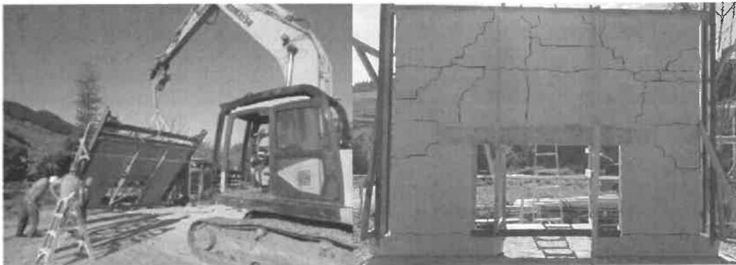
Figure 2: Adobe veneer wall panel 4m x 3m with lintel, a) tilt test at about 45 degrees, b) highlighted crack pattern following all tests. Photos: Hugh Morris
