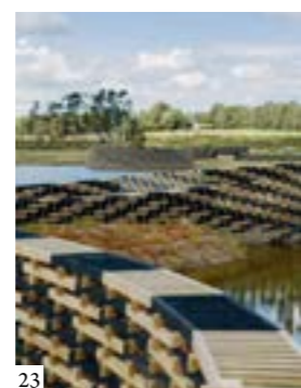
Figure 24 Weaving pattern of river walls constructed with timber
